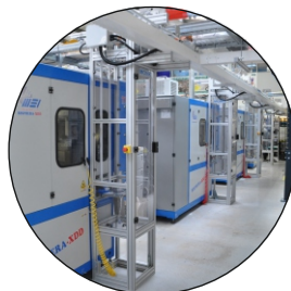
Lifts to Overhead Conveyors
